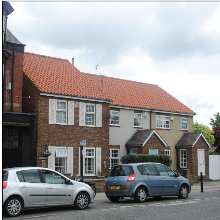
Photo 8. Nos 40-42a Front Street
