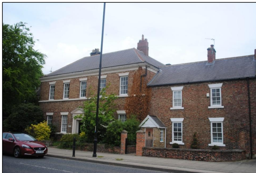
Photo 7. Boldon House & 64 Front Street
